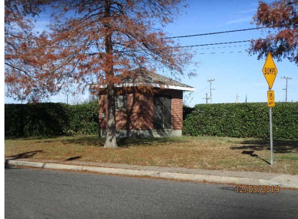
Photograph 18. View of the on-site pump house.
