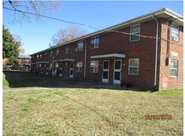
Photograph 2. View of the rear of the typical residential building.
